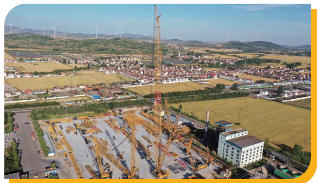
Overall Crane Testing
